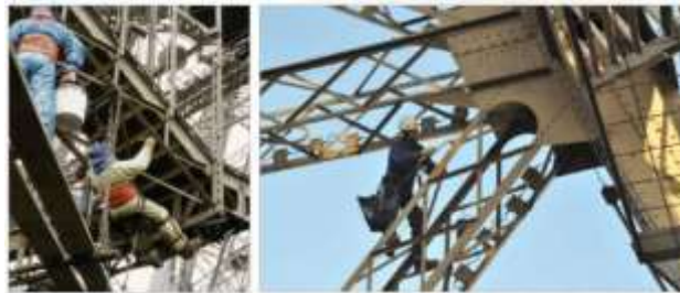
Figure (12): maintenance of Eiffel Tower
