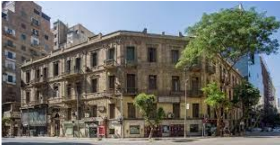
Figure 11: La viennoise building before development in 2015
