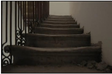
Figure 13: Main stair before development
