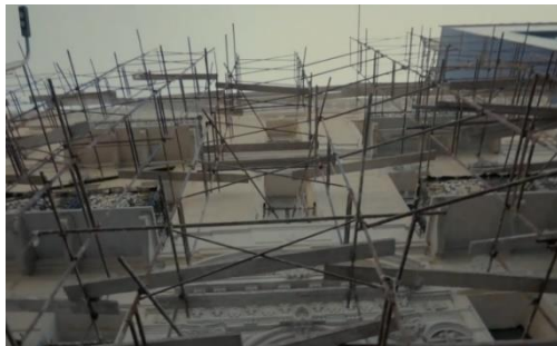
Figure 17: External facade development work
