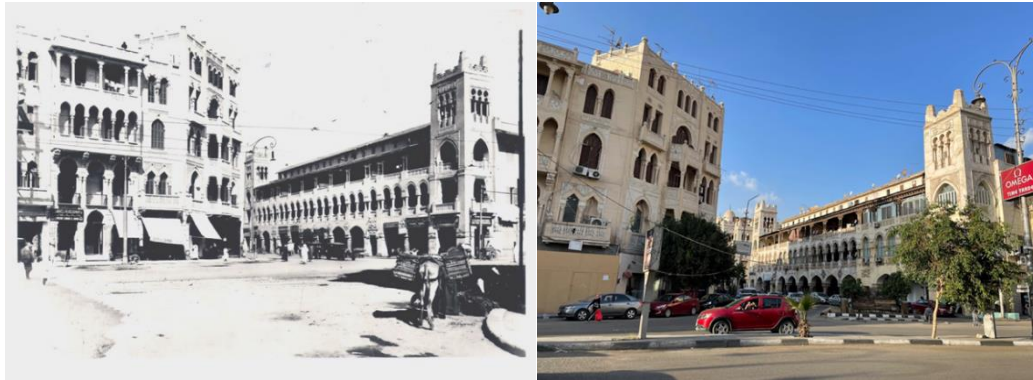
Fig. 4: Boulevard Ibrahim El-Lakkani. Top: 1920s [7, p. 58] and Bottom: 2021 (taken by author)
