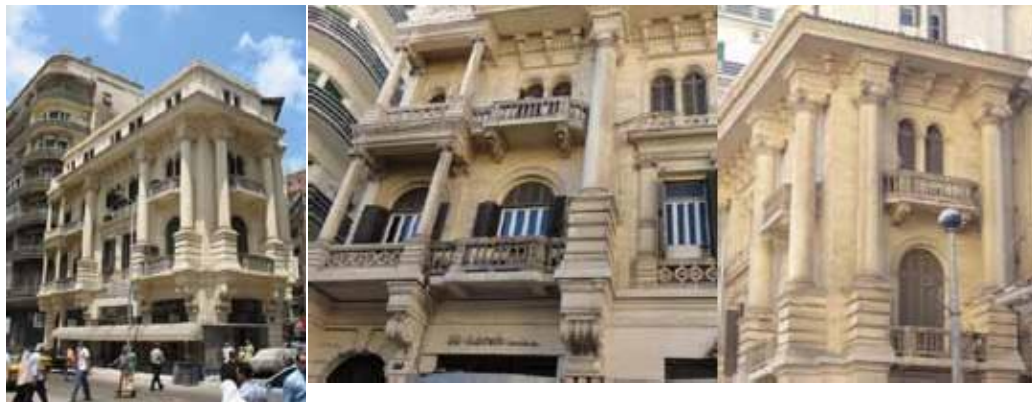
Fig. 2 : Ornamental details of a High Eclectic Mannerist building; with a mix of different styles; plain shaft Ionic columns and pilasters, egg and dart motifs resembling life and death, cornice with dentils, variety of bracket ornaments some with animals heads and some with acanthus leaves others with voluted form, balcony balustrades with columns and scroll
