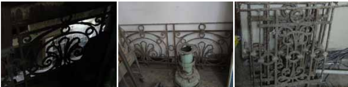
Fig. 12: Ornamental detail of forged iron (fer forge) balcony grills with scrolls, circular and anthemion leaf patterns, wide spread classical rhythmical repetition of classical motifs.(Residential building in Fouad St.)
