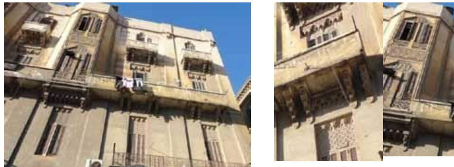
Fig. 4: Ornamental details of a Neo Islamic residential building with traditional elements of Islamic ornaments; Stalactites and brackets beneath balconies, panels
