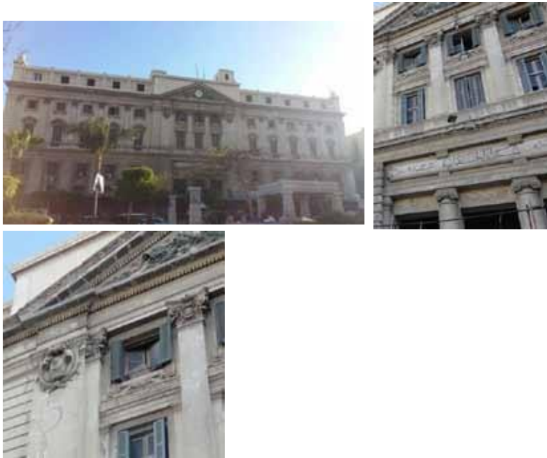
Fig. 3 : Ornamental details of a Neo classic style court house; symmetrical façade with triangular pediment containing classical motifs of foliage, plain shaft Ionic columns with voluted capitals with egg and dart motifs, composite pedestals, third storey level windows have a pediment, stone effect walls, classical balcony balustrades. (Manshieh square District)
