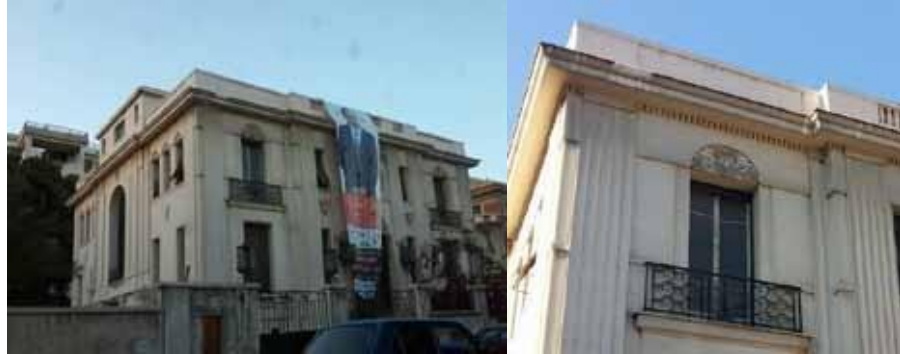
Fig.13 : Ornamental details of an Art Deco Style villa facades, with a mix of different styles; vertical pilasters with shallow volutes and a minimal capital, accentuates gracefulness of lines, semicircular panels over windows and doors with decorative bas relief ornaments of gargoyles heads and geometric repeated patterns of foliage like motifs, dentil ornament surrounding the top, gargoyles heads symbolizing guardians, forged iron (fer forge) balcony grills with scroll patterns, classical balustrades on parts of the parapet. (Soliman Yousri St.- Latin District)
