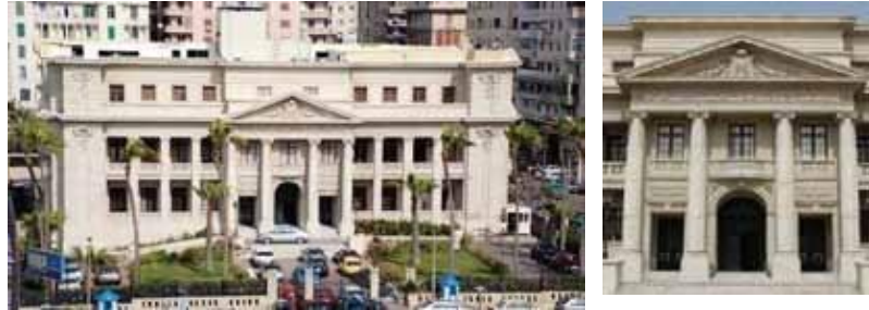
Fig.7 : Ornamental details of a Greek Revival Style villa; the main entrance accentuated with triangular pediment and entablature with classical motifs, a metope and triglyph frieze also dentils, four Ionic columns with pedestals, walls with stone effect, Greek geometric patterned balcony grills, side broken pediments centered with circular wreath with laurel leaves. (Raml District, Cournich Road) (villa now: Women public service center)
