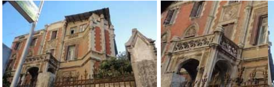
Fig. 9: Ornamental details of a Gothic revival style villa facade; with a porch of gothic columns, vertical gothic pilasters, gothic pointed transom over the entrance, a label around windows, balconies grills and parapet with gothic ornaments, quoins on corner sides, rectangular and flattened pointed arches panels with gothic bas relief motifs, urns on top edges. (Latin District)
